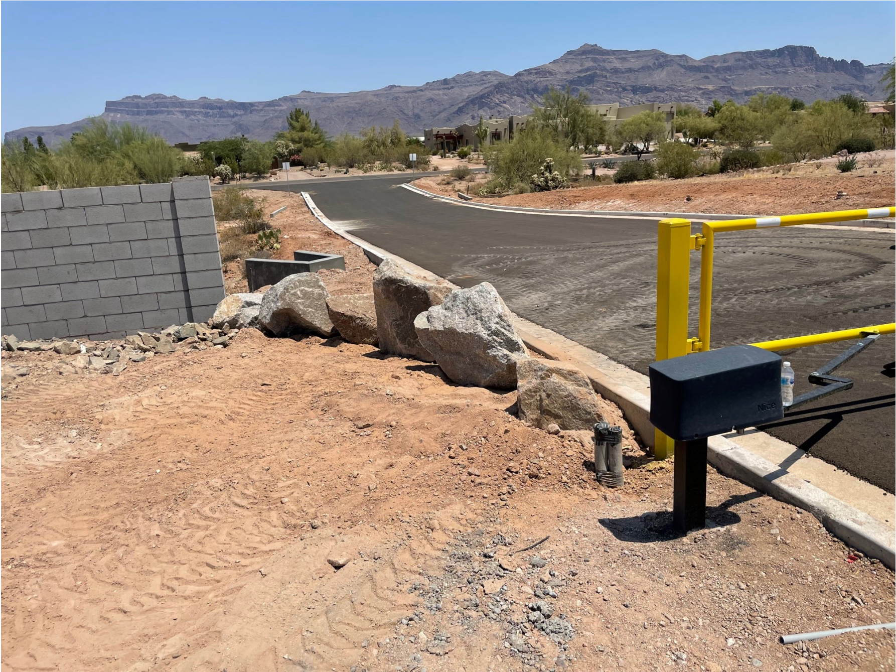
Pic 7- west side of gate, boulders/landscape installed by developer
