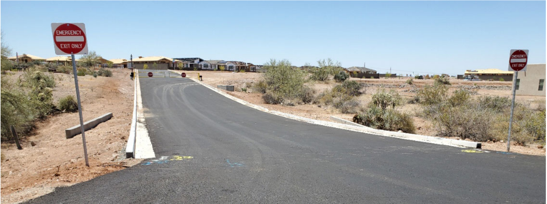
Pic 2- same as Pic 1, gate in the closed position
