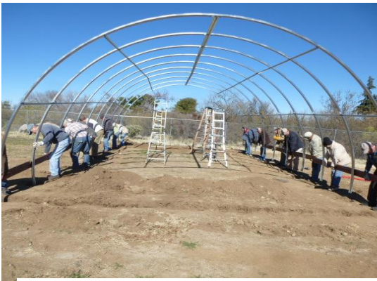
Volunteers erecting a hoop house
