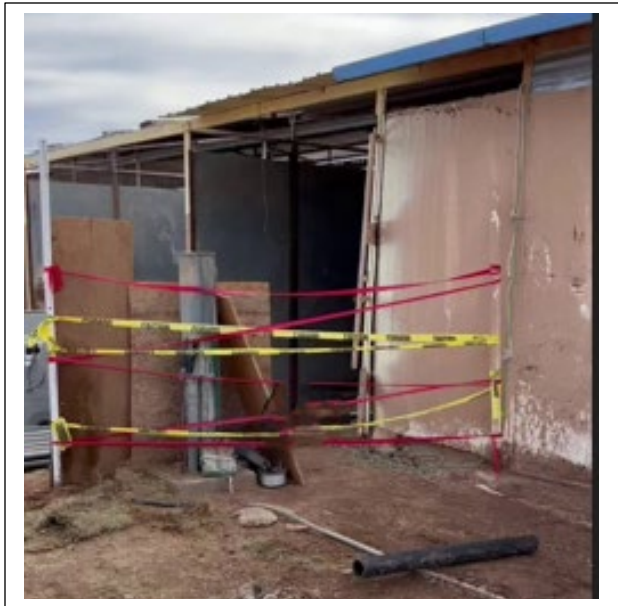
Old Pedestal – Removed
