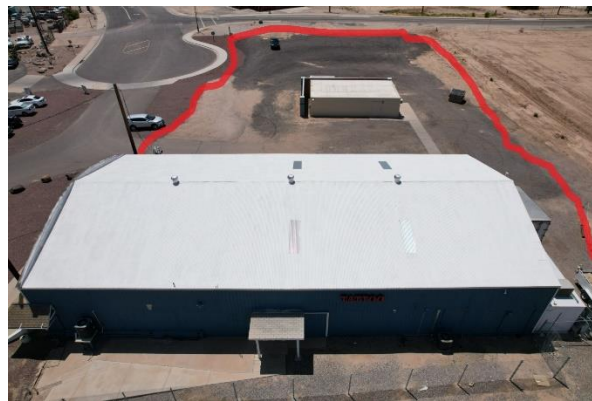
Red line defines parking lot area to be completed.
