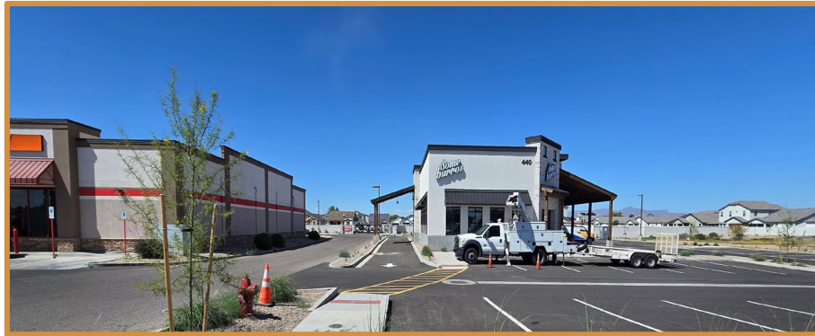
Looking North onto site
