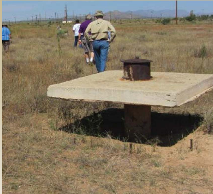
Subsidence, leaving Well head exposed above ground
